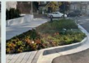
Green Infrastructure Curb Bulge
