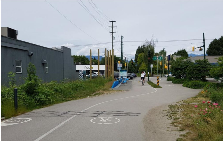
Figure 5a Arbutus Trail - curved (bend-out) alignment at signalized intersection approach to major street (Note separated bike and pedestrian lanes)
