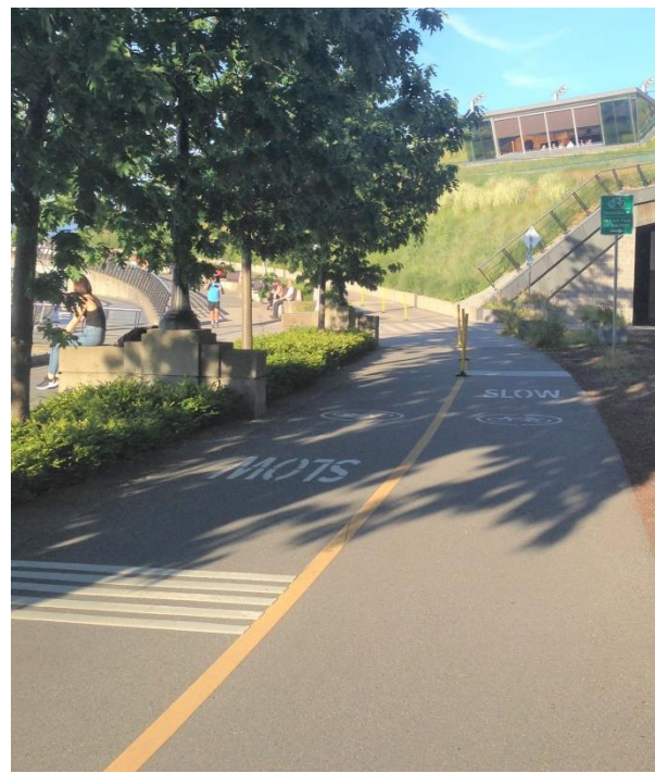
Figure 6b Coal Harbour Bike Trail – Slow Zone. Note rumble strips, markings and flexi-posts
