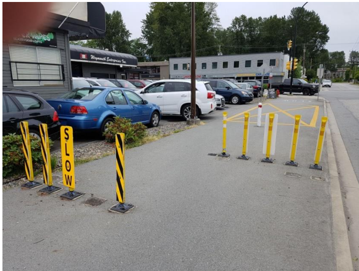
Figure 7 Spirit Trail near Pemberton Ave, North Vancouver (looking east) – existing baffle gate as modified by DNV to permit traverse by larger vehicles.
