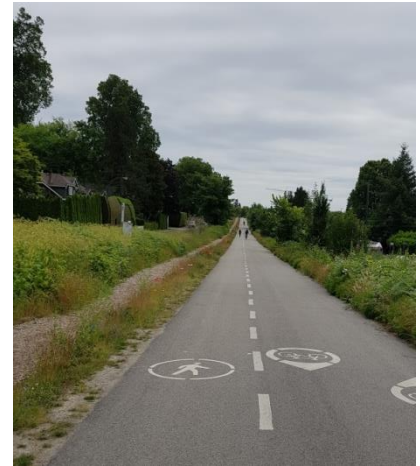
Figure 5b Arbutus Trail Note separated asymmetric pedestrian and (two-way) bike lanes and adjacent wood chip running path
