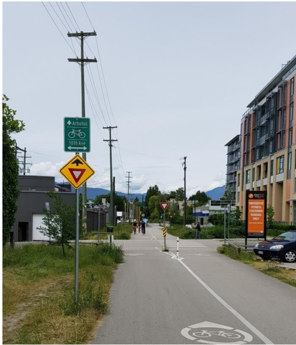
Figure 6a Arbutus MU Trail – Yield control at minor street intersection without stop lines
