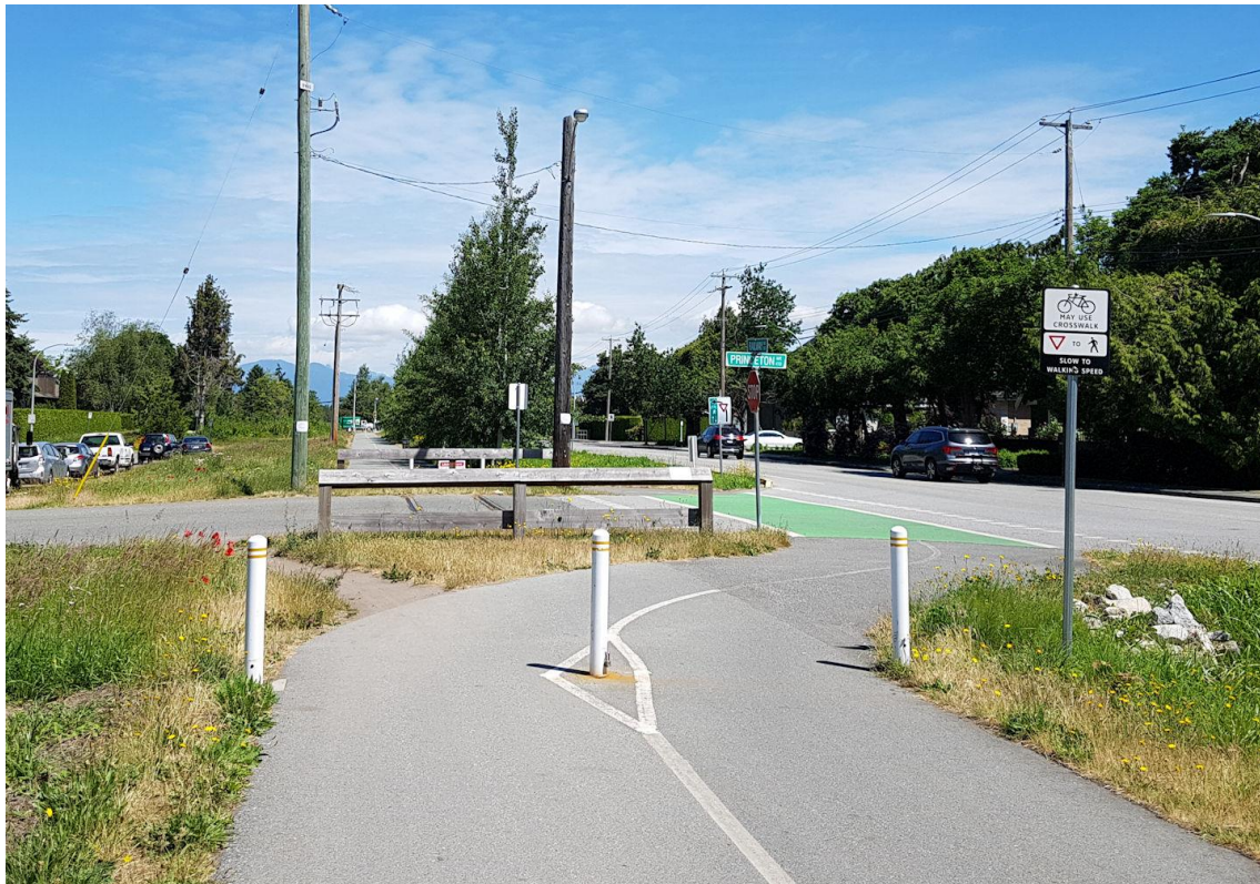
Figure 5c Railway Trail - curved (bend in) alignment at intersection approach to minor street with stop line (Note separated directional MU lanes with bollards; green painted crossing; and bike crossing permit and yield to pedestrians signs)
