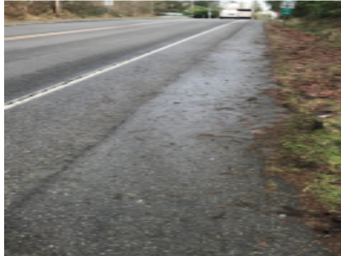
Figure 1.12 From the east end of the south side fence to 216 Street the bike/pedestrian pathway is at travel lane level and 163 cm wide.
