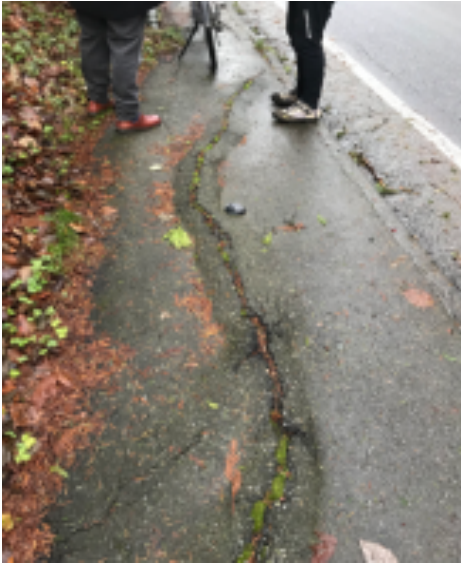
Figure 1.5 Sidewalk on southside of 40 Avenue.
