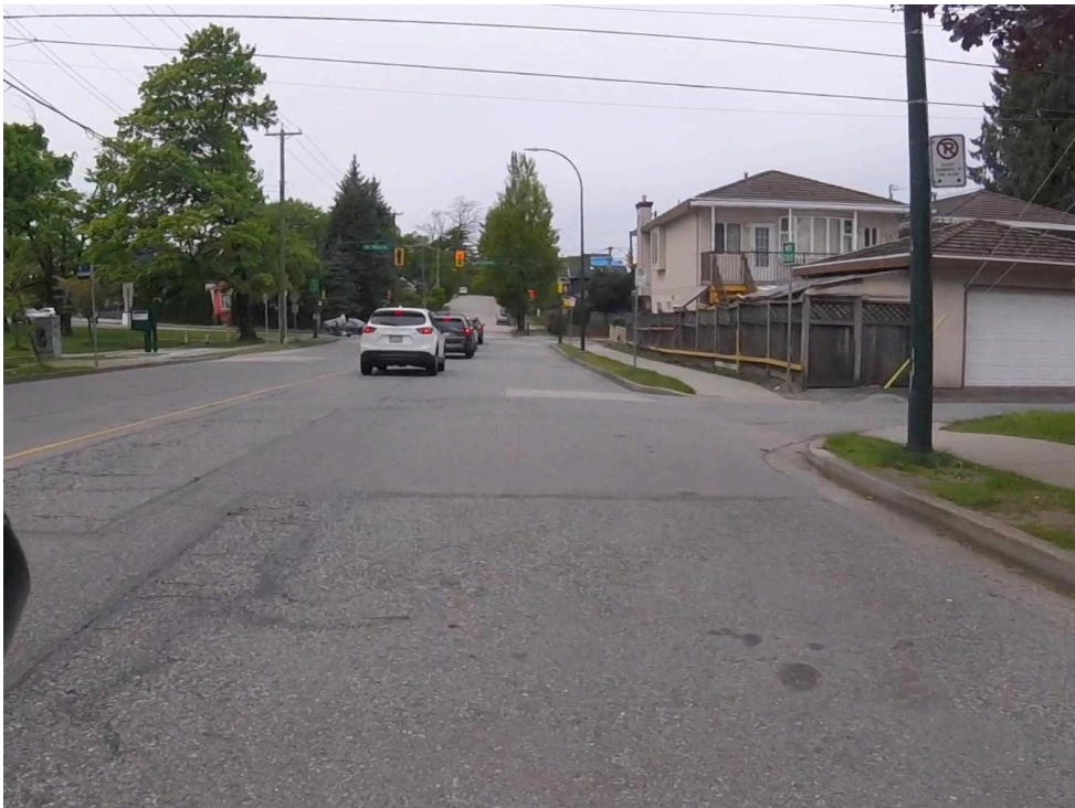
Figure 8 - 29th Ave from the Skytrain station west to Slocan St.
