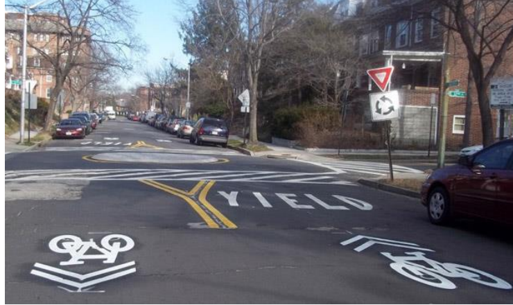
Figure 1 Traffic calmed street with raised intersection and mini traffic circle in Baltimore, MD
