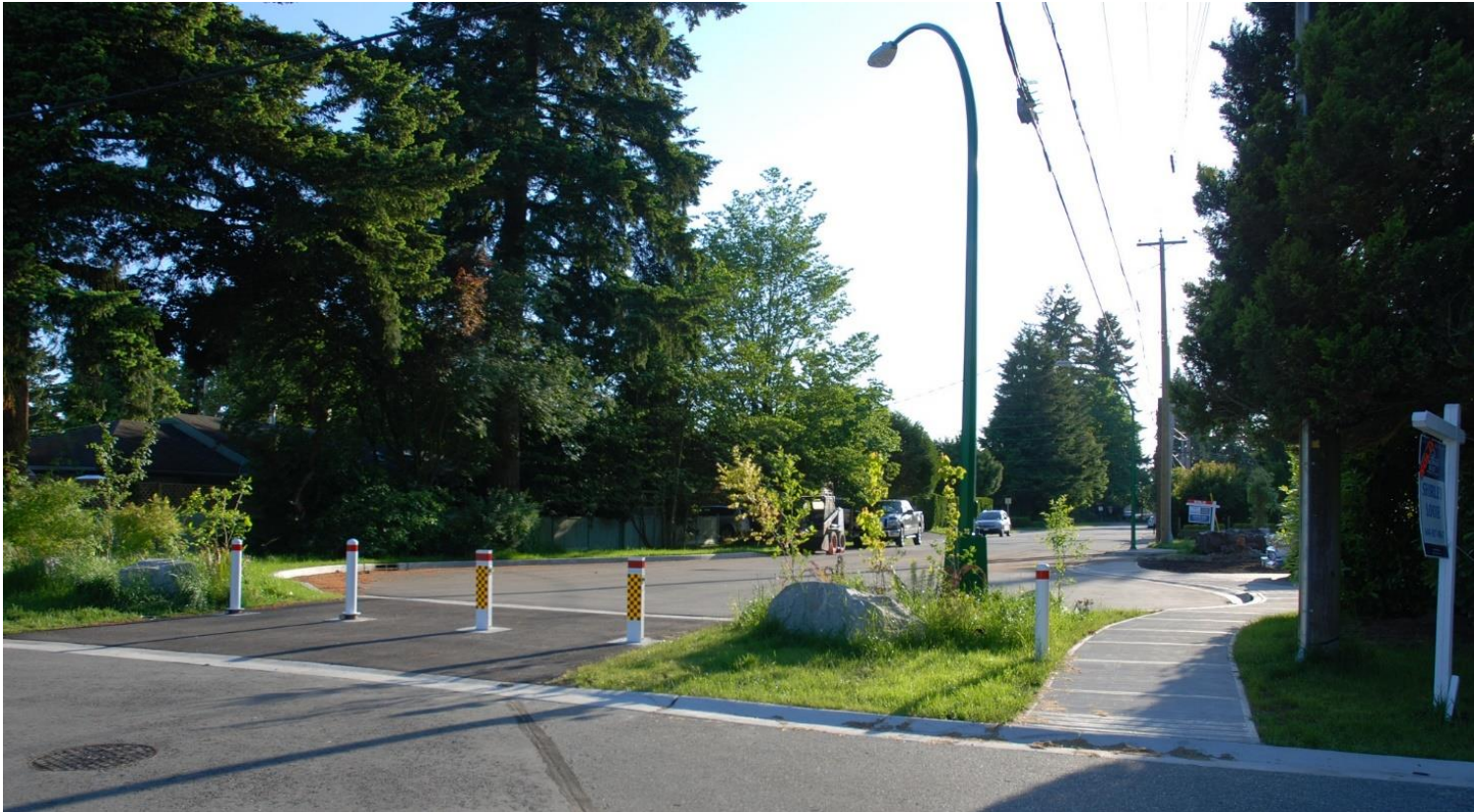
Traffic diverter on Hope Road
