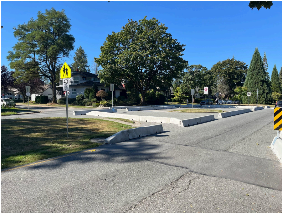
Figure 2 - Unmarked crossing at the eastern end of the gravity barriers on 16th Ave at Wallace
