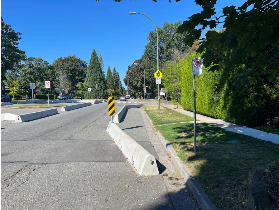
Figure 5 - Gravity Barriers on 16th Ave westbound at Wallace have no accommodation for people cycling
