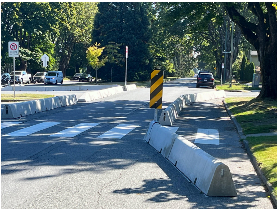
Figure 6 - Gravity Barriers on 16th Ave eastbound at Wallace have no accommodation for people cycling
