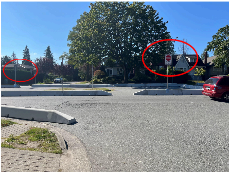
Figure 4 - Openings have been left in the gravity barriers for people cycling to cross, but these are marked at only two points; they are aligned with the centrelines of Wallace St. north and south; and they allow diagonal crossings.
