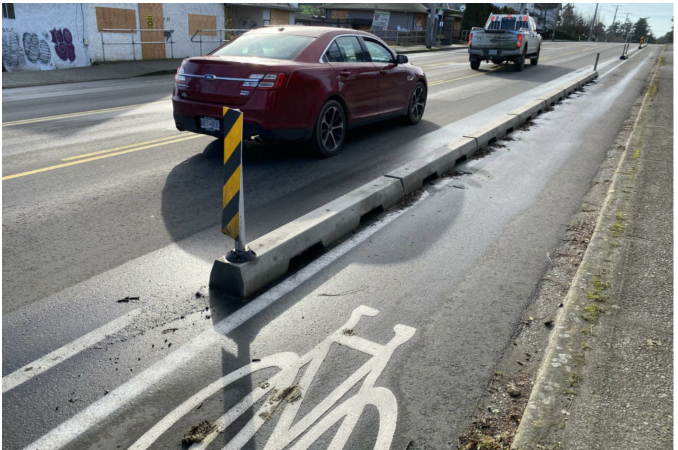
Figure 2 - Prefabricated curbs used to provide quick-build, low-cost bike lanes on Tillicum Road in Saanich. Photo courtesy Chris Campbell.
