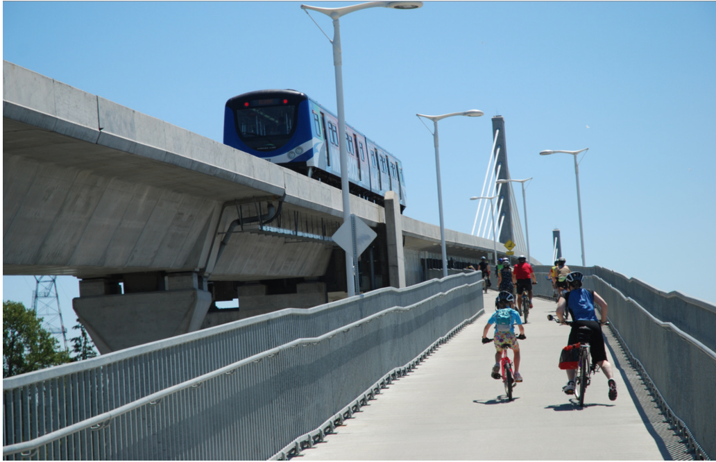
Canada Line Bridge
