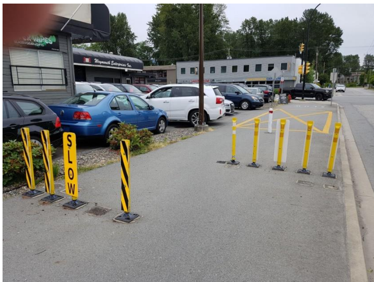
Figure 6 Spirit Trail near Pemberton Ave, North Vancouver (looking east) – existing baffle gate as modified by DNV to permit traverse by larger vehicles.
