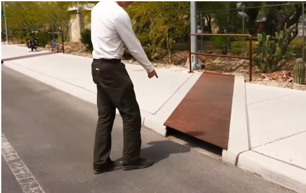
Example of a drainage trough in Phoenix, Arizona that leads to a drainage swale.
