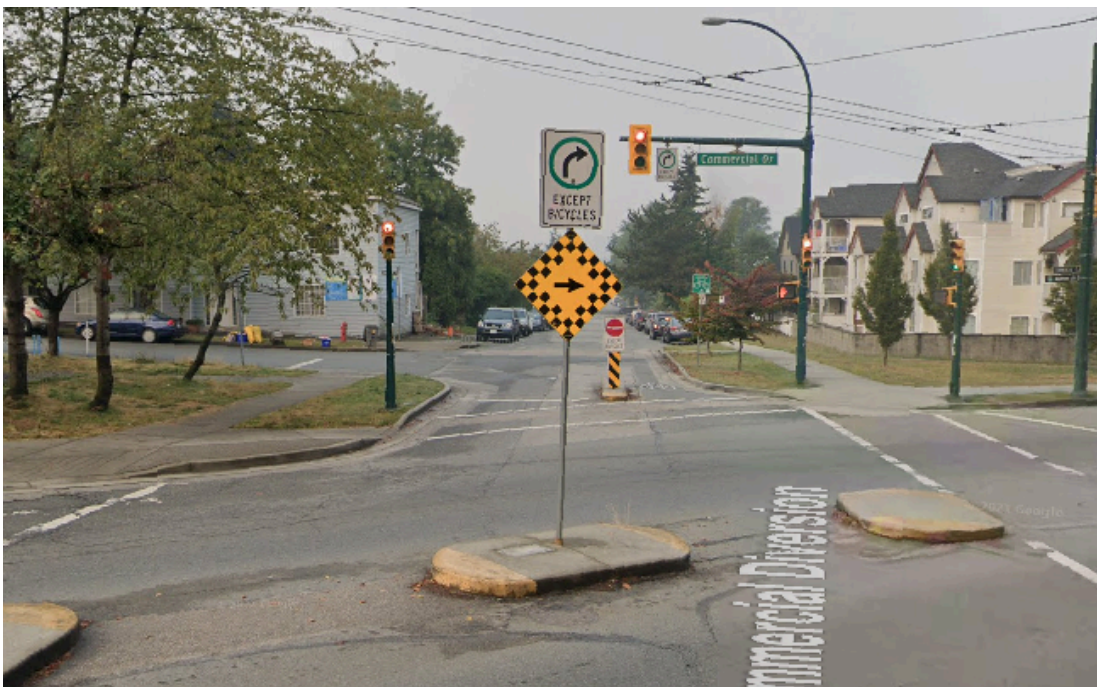
Figure 1 - Adanac Street at Commercial Drive, Vancouver. The traffic diverter lowers vehicle volumes, ensuring more safety for people biking. Courtesy Google Maps.
