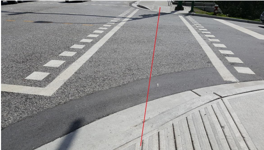
Crossbike on Bewicke Looking East
