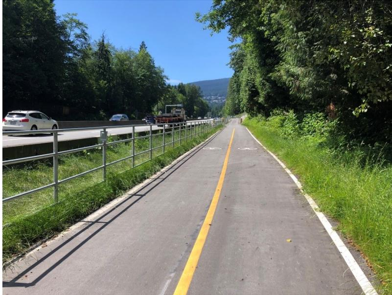
**The design of the Hugo Ray connector along Highway 1 in West Vancouver is a good model for cycle highways. It is separated and protected from Highway traffic and is wide enough for users to pass safely. Where pedestrian use is higher, cycling and walking paths should be separated.**
