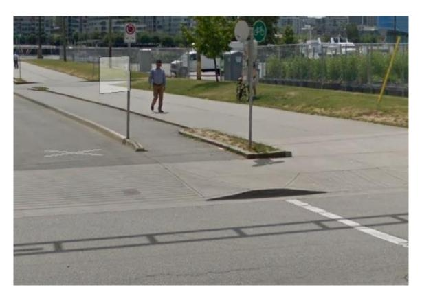
Maintenance to Ontario protected lanes 49<sup>th</sup> -52<sup>nd</sup>, including sweeping and realigning gravity barriers
