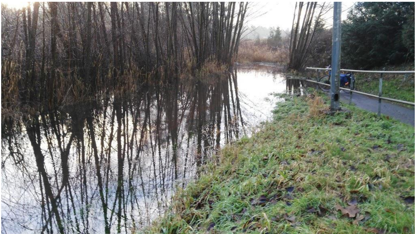
Photo Location 2 - Flooding on path
