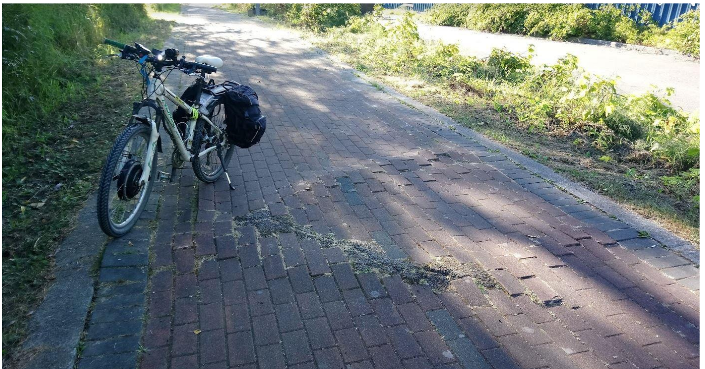
Photo Location 4 - Heaved bricks on path
