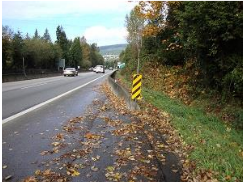
Figure 4: Looking west, east of 3 rd Street. Proposed bike path would be to the right of no-post barrier.
