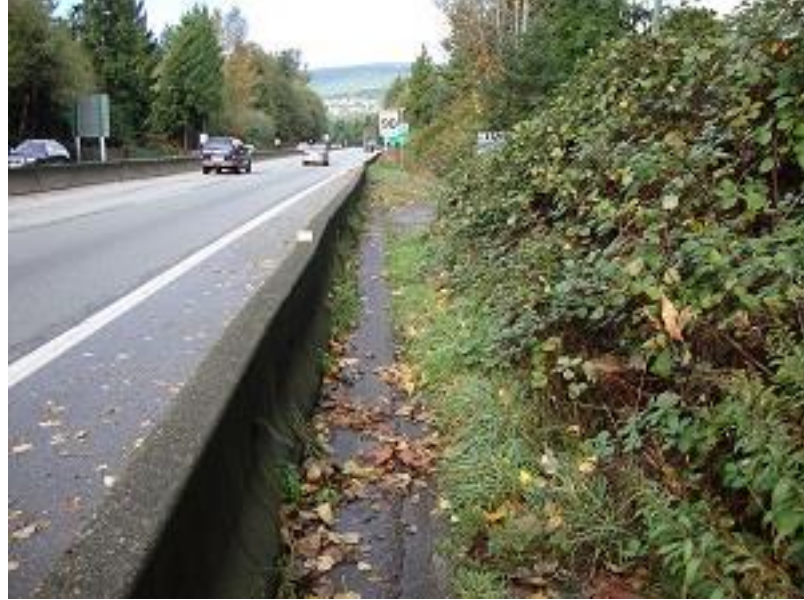
Figure 5: Looking west, current space behind no-post barrier near 3 rd Street
