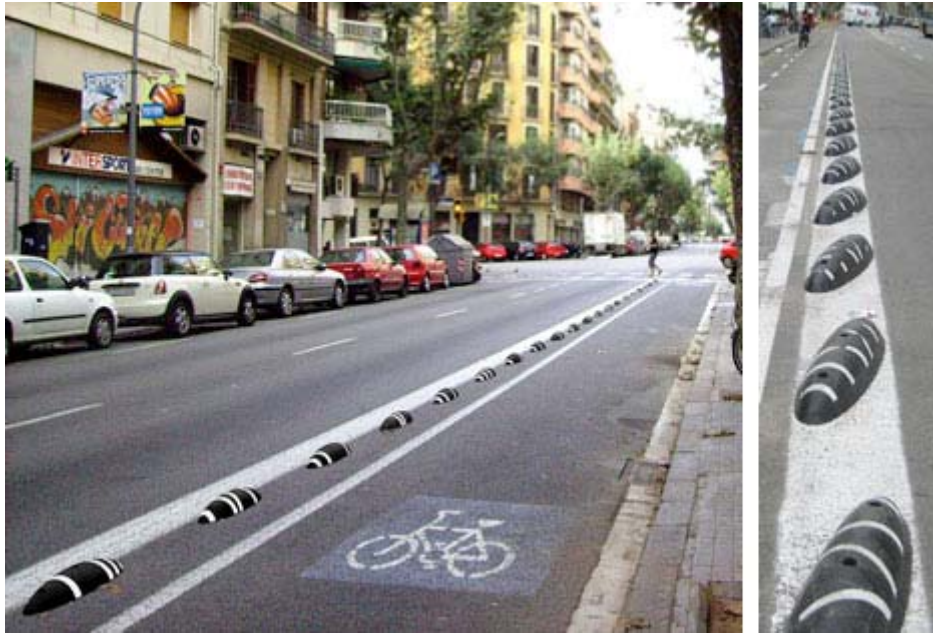
Figure 3. Example of a physical barrier that allows emergency vehicle access
