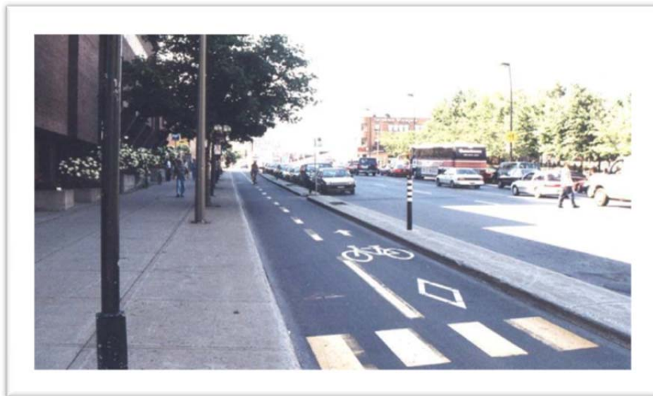
Figure 2. Example of a physical barrier that allows emergency vehicle access
