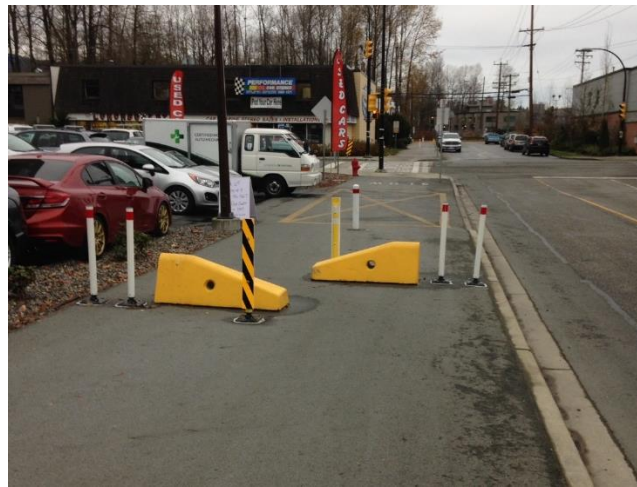
Figure 1: Baffle on Spirit Trail near Pemberton Avenue
