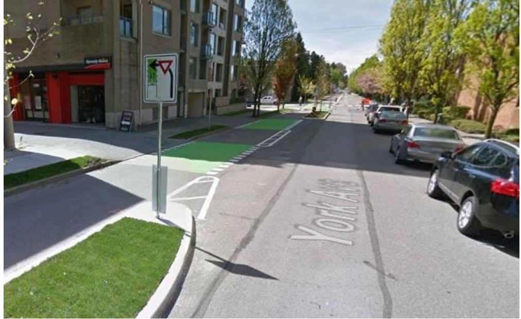
Figure 6: Green marking at lane and driveway crossings to alert drivers and cyclists (York Street, City of Vancouver)
