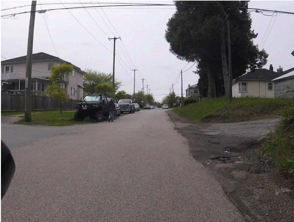
Figure 7 - The north end of the proposed Kerr St Bikeway along Skeena St
