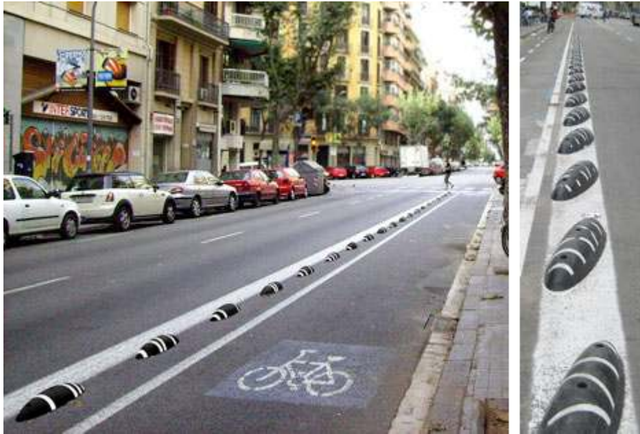
Figure 3. Example of a physical barrier that does not prevent emergency vehicle access
