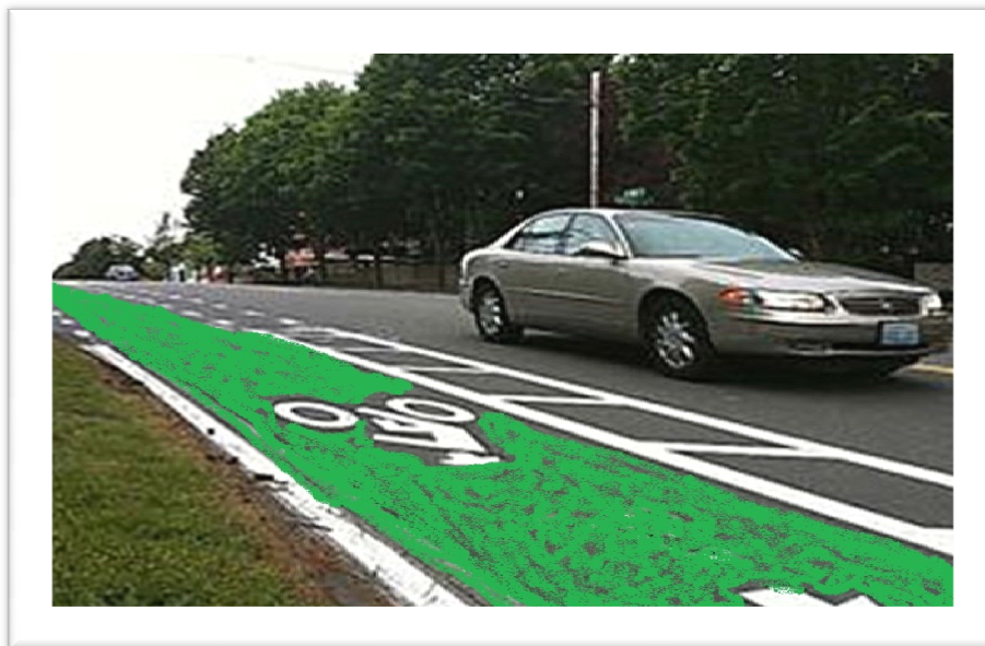
Figure 4. Separation Stripe and Green Lane
