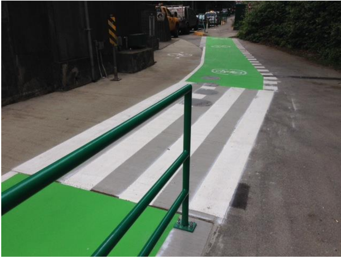
Figure 3: Clearly marked pedestrian and cycling areas in high conflict zone at Lions Gate Bridge near Prospect Point. Cycling speeds are high downhill from the bridge while tourists walk through this area to view the bridge.
