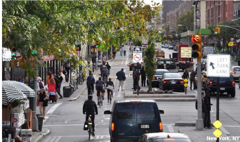
Figure 9: Example of protected bike lane on shopping street (New York City)
