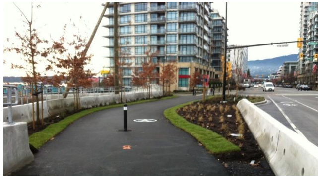
Figure 1: Unnecessary and hazardous bollard on Spirit Trail at Esplanade
