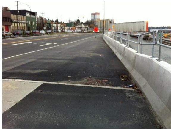
Figure 3: Hazardous curb on Spirit Trail at Esplanade
