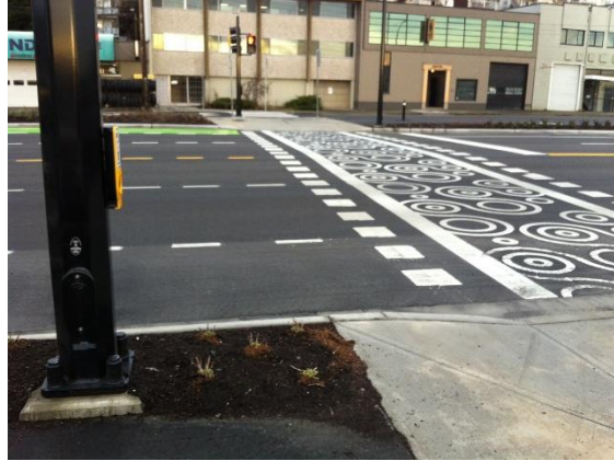
Figure 6: Push button at Spirit Trail crossing of Esplanade
