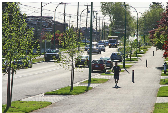
Multiple driveways and rigid bollards along the Rumble Street multi-use pathway
