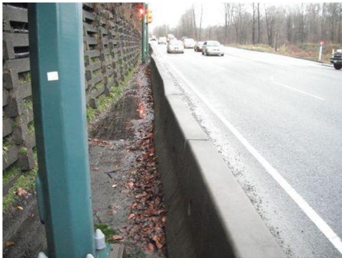
Looking north along Lougheed towards the intersection.
