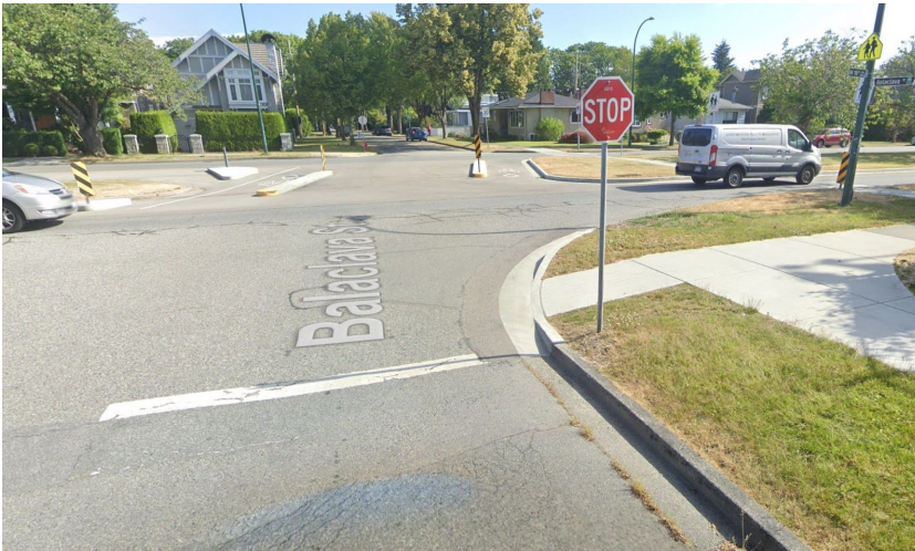
Figure 4: Bikeway crossing 16th Ave with new curbs
