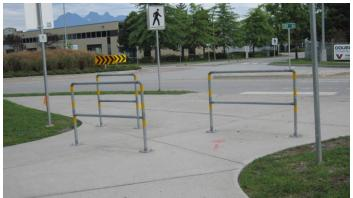
• A set of two bollards spaced less than 90 cm apart has been installed on each of the immediate approach and departure to the bridge sidewalks. These bollards are improperly located, spaced and marked. One of our members suffered serious bruising when crashing into one of the improperly placed bollards. We question the need for both baffles and bollards at this location. Surely one or the other, properly designed in accordance with contemporary guidelines, would suffice.
