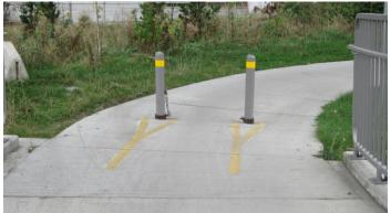
• The ramps that provide cycling access to and from the bridge paths on the north side appear to have been designed as "sidewalk crossings" (i.e., reinforced, ramped sidewalk sections designed for the passage of motor vehicles). These are less than ideal for cyclists transitioning from the bridge path to the roadway shoulder and hazardous for cyclists transitioning from the roadway
