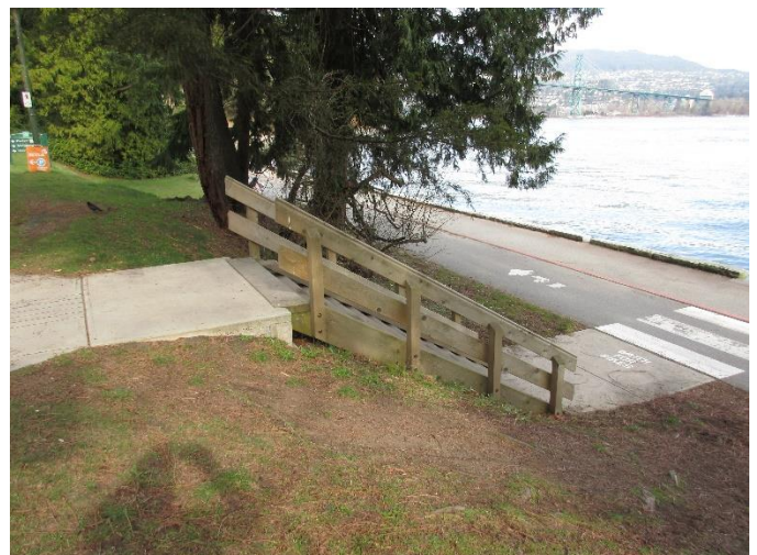
Figure 2 - Staircase built in lieu of the recommended ramp
