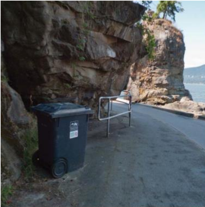
A blind corner with a pinch point at Siwash Rock. The existing post and rail fence should be replaced as it can "snag" handlebars.
