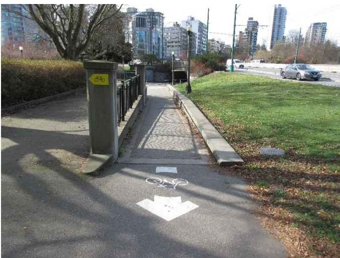
Figure 7 - Dangerously narrow Multi Use Path
