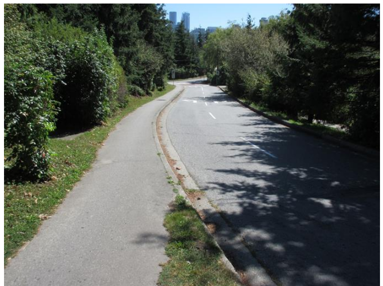
Figure 11 - Existing paved path that replaces the need for 8b
