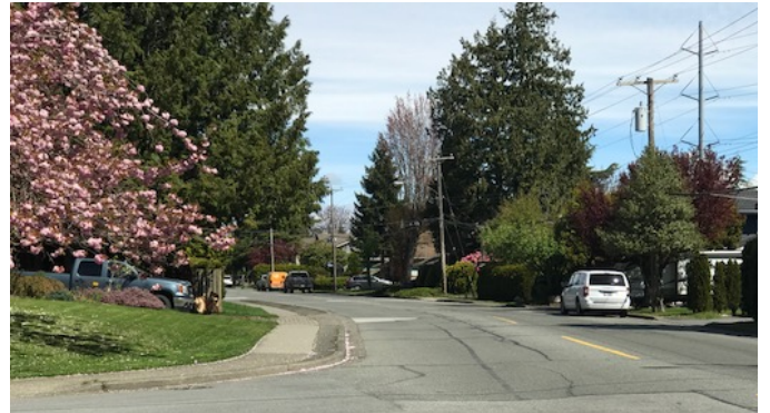
53A St, looking north at Camaro Drive
