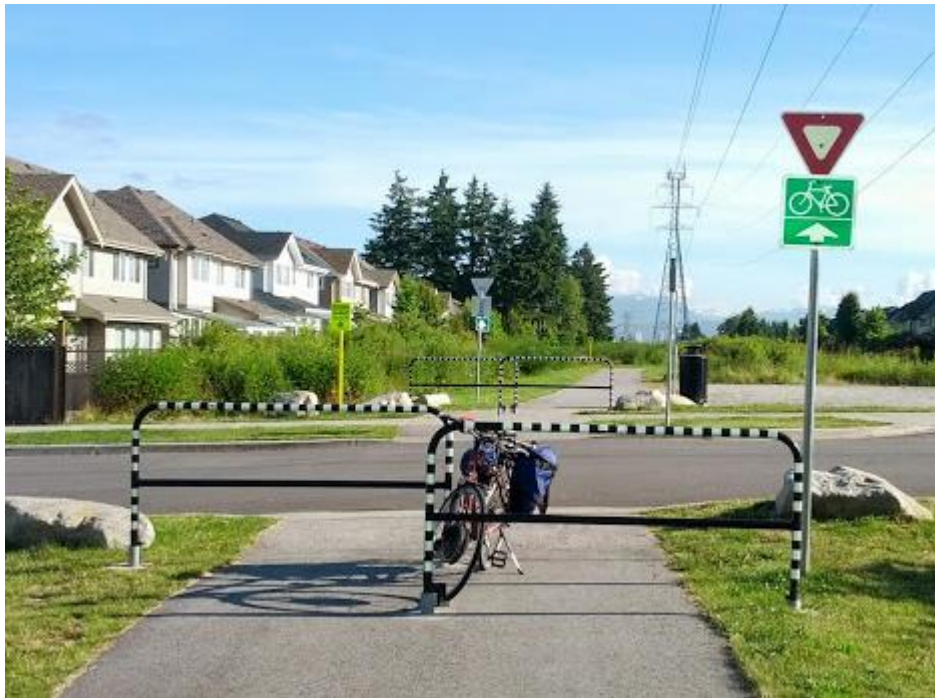
Typical new greenway crossing in North Delta. Does not warn drivers of a crosswalk, baffle gates restrict passage of bike trailers, restrict vehicle access. Location is at 82 nd Avenue near 108 th Street
