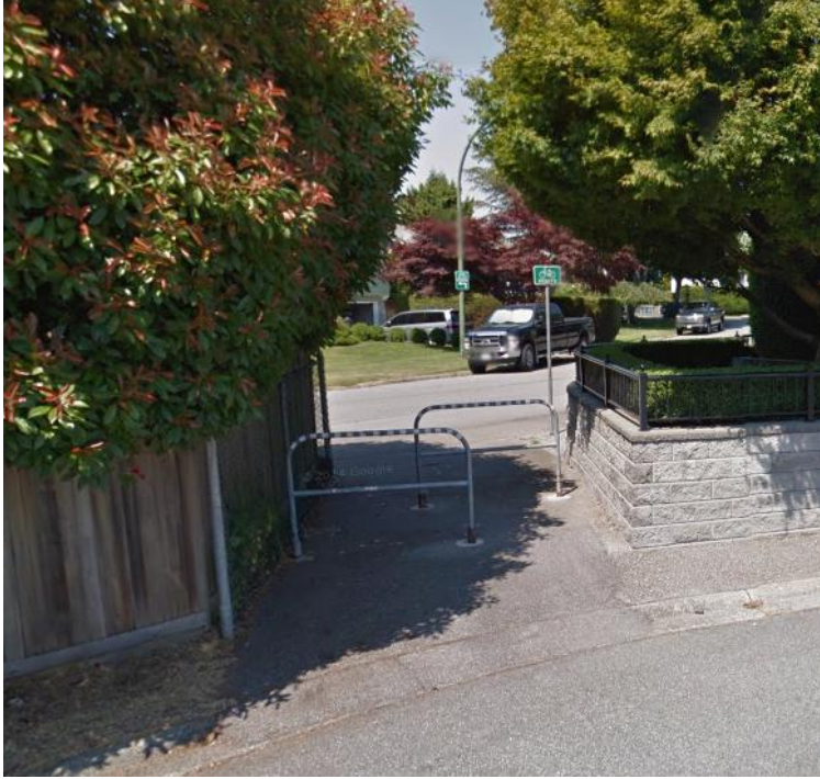
Cory Drive to Caribou Road path – Access is difficult for regular bikes due to the very narrow openings
