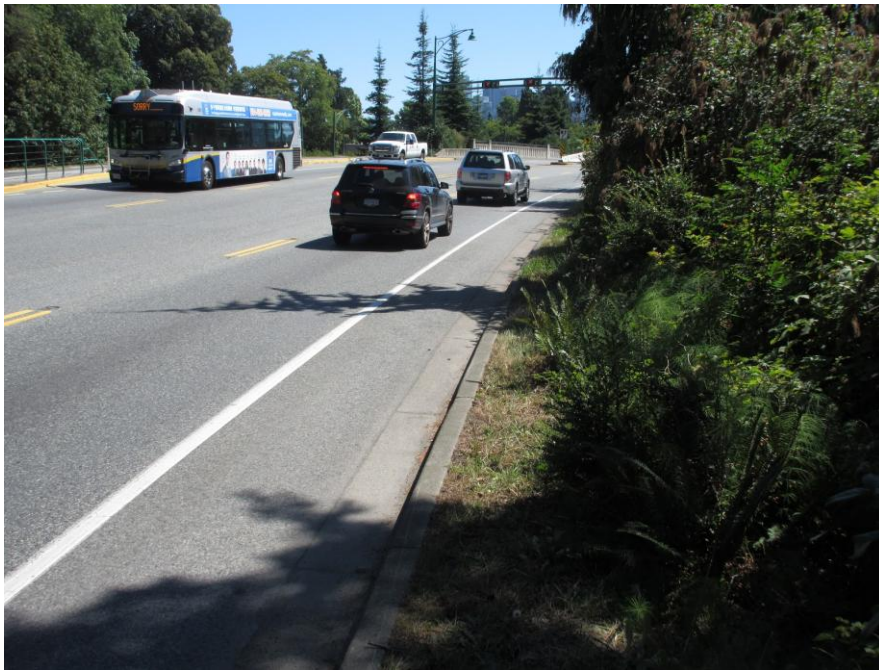
Figure 3 - Causeway southbound (west) - Unprotected painted bicycle lane
