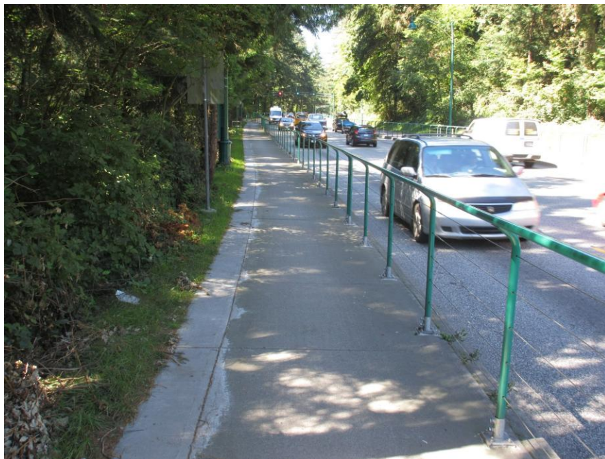
Figure 2 - Causeway southbound (west) bicycle path
