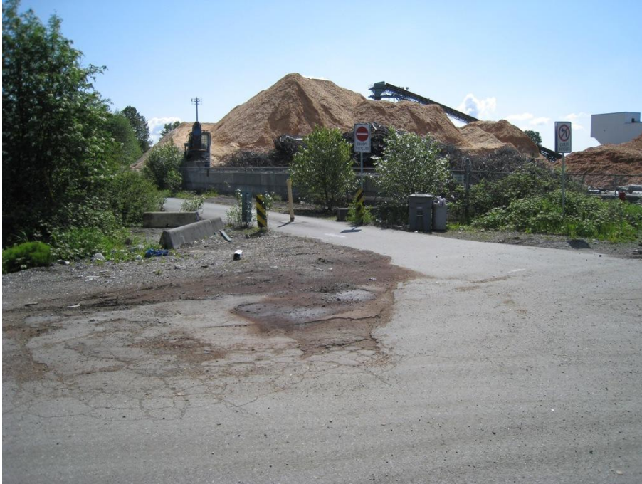
Figure 12 - The entrances to and exits from the current separated cycle paths along the Kent Ave South ROW require wayfinding signage to direct people on bikes. The route is not intuitive here.
