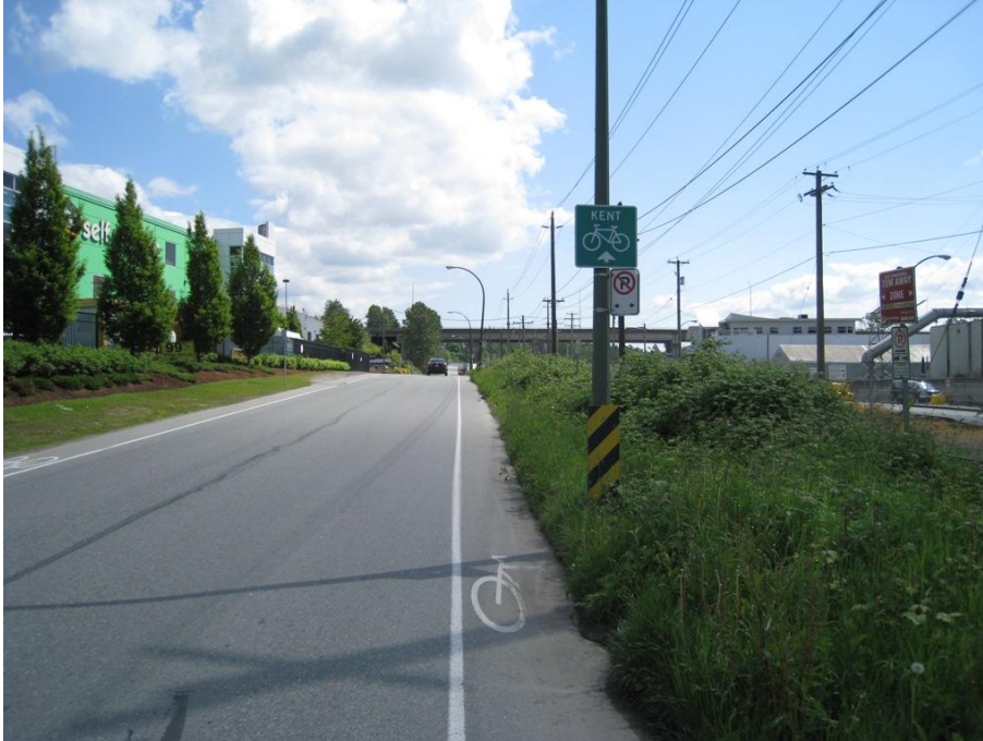
Figure 14 - The existing shoulder bicycle lane along Kent Ave. North near the Knight Street Bridge is not wide enough for a standard bicycle stencil, let alone comfortable and safe for most people cycling.
