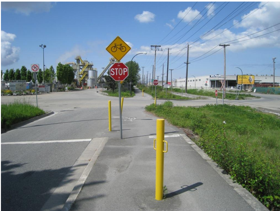
Figure 13 - Bollards are not well places and create a crash hazard, particularly at night. Concrete barriers would provide additional protection from motor vehicles after the first stop sign, to the intersection.
