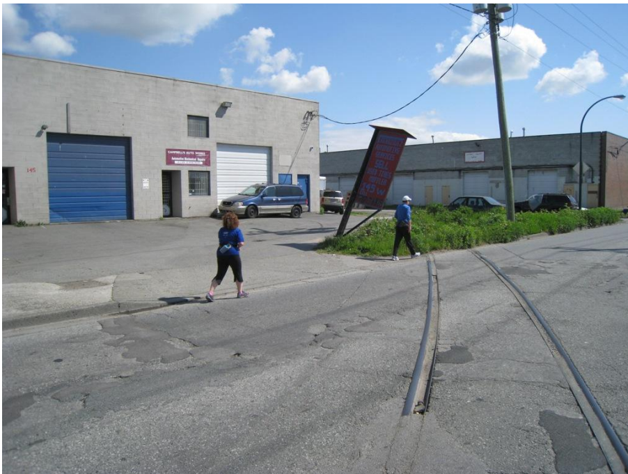
Figure 11 - Abandoned railway tracks are particularly dangerous when the tracks cross the roadway at oblique angles that can catch a bicycle wheel and create a risk of falling into vehicle traffic.
