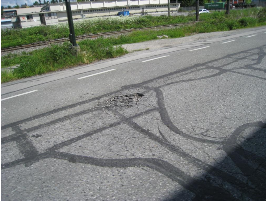
Figure 10 - Poor quality pavement exists in many sections, particularly along the edges of the roadway where people on bikes usually travel.
