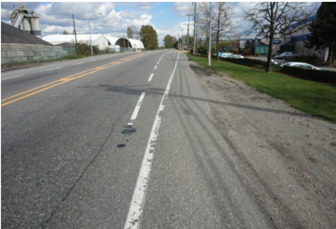
Another example where better lane marking is needed at River Road and 82nd Street:
