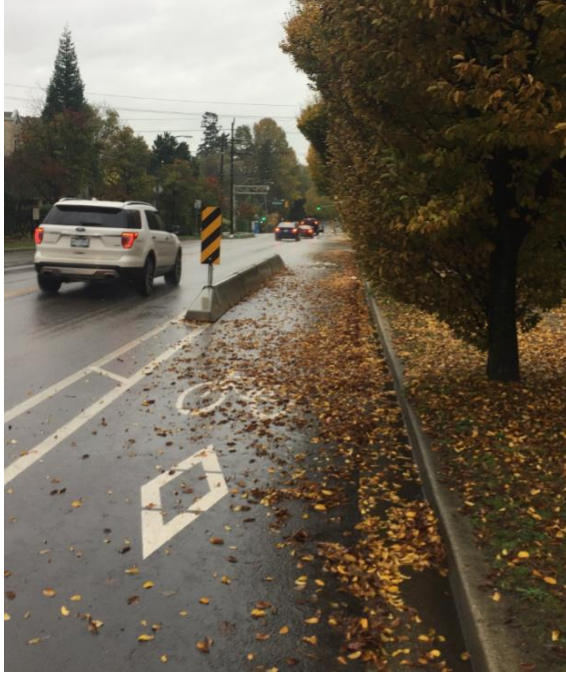
Figure 29: Trees Obstructing the Bicycle Lane
