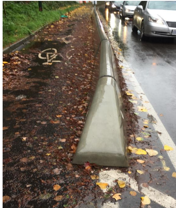
Figure 11: Shifting Concrete Barriers
