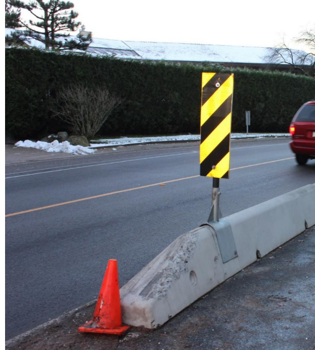
Figure 14: Example of a Traffic Cone Added in Front of Barrier to Increase Barrier Visibility
