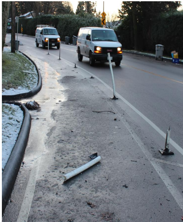
Figure 12: Damage to Plastic Bollards
