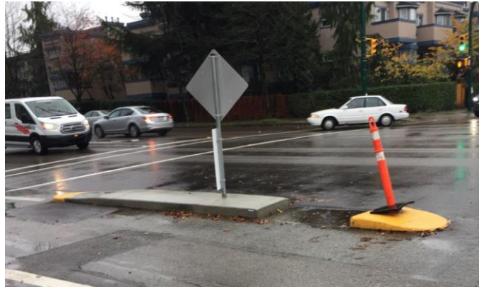
Figure 15: Example of Yellow Paint Used to Enhance Visibility
