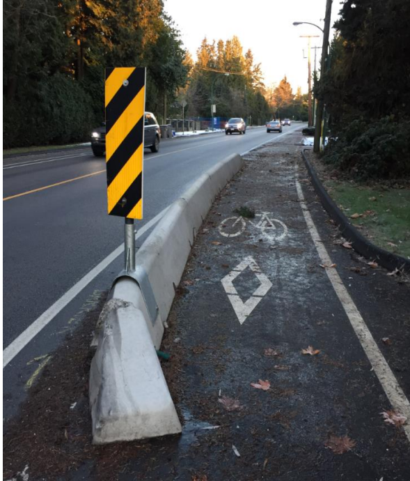
Figure 13: Broken and Scuffed Concrete Barriers
