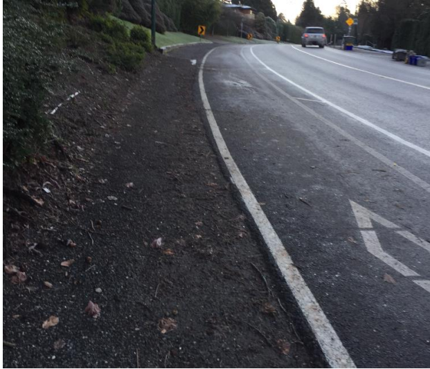
Figure 10: Example of White Lane Line Adjacent to the Edge of the Asphalt
