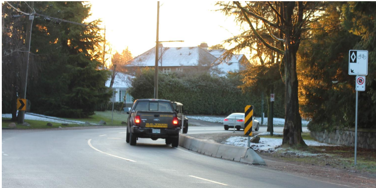
Figure 20: Vehicle Encroaching into the Concrete Barrier While Navigating a Curve in the Road
