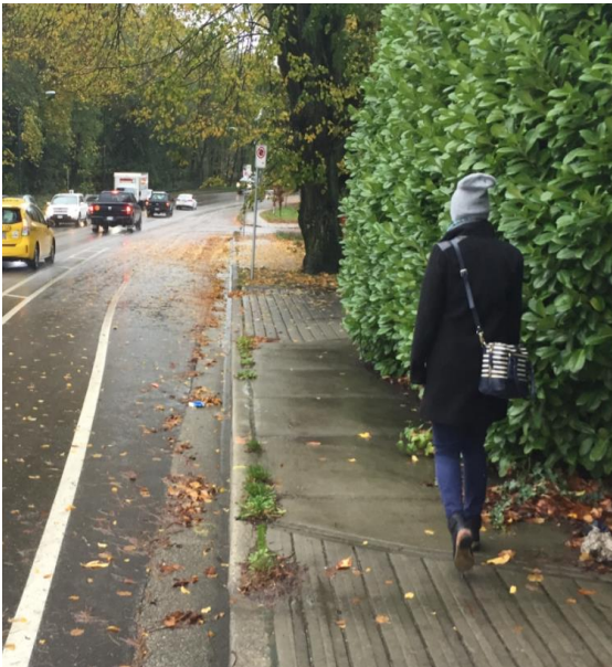
Figure 23: Overgrown Vegetation Adjacent to Sidewalk
