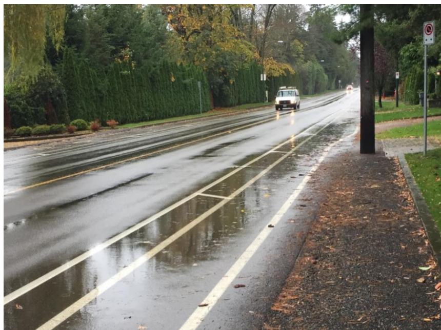
Figure 8: Example of a Location Where the Width of The Bicycle Lane is Below 1.5 Metres
