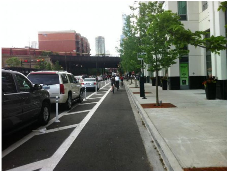
Figure 2 - Example cheap parking protected bike lane with delineator posts
