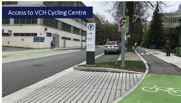
Figure 35. Access to VCH Cycling Centre is awkward for westbound cyclists; Cycling Centre door also opens directly into the pedestrian space (access has since been modified by VCH Cycling Centre)
