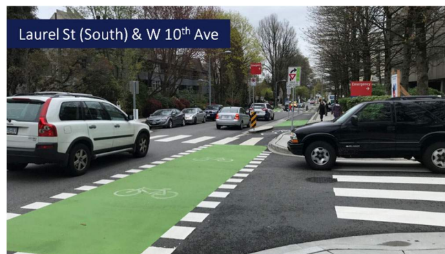
Figure 33. Difficult for paramedics driving ambulances turning right into the Emergency entrance to see cyclists headed eastbound in protected bike lane
