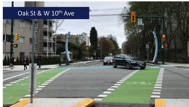
Figure 32. Lack of notice for eastbound pedestrians and cyclists of leading protected left phase for the east approach
