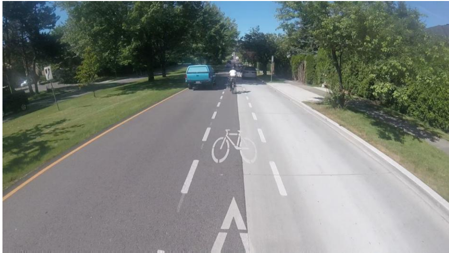
Figure 5 - Bus pad creates a dangerous pavement seam
