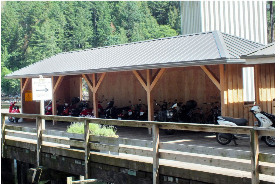
Reference Photo 2 - Example of a short-term bike parking facility at Snug Cove, Bowen Island
