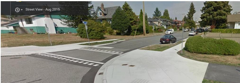
**Figure 1: Multi-use path crosswalk with elephant's feet on Jones Ave at 16<sup>th</sup> St**
