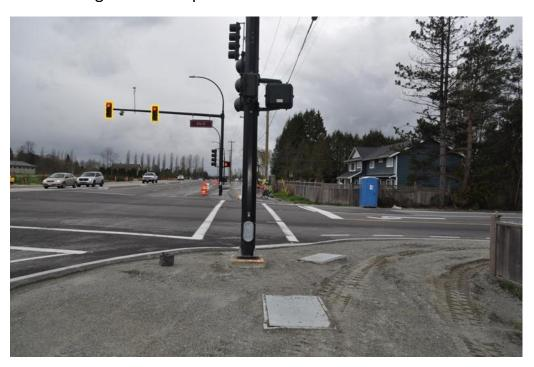
The path that has already been paved on the west side of the intersection does not line up with the crossing nor with the let-down on the east side:
