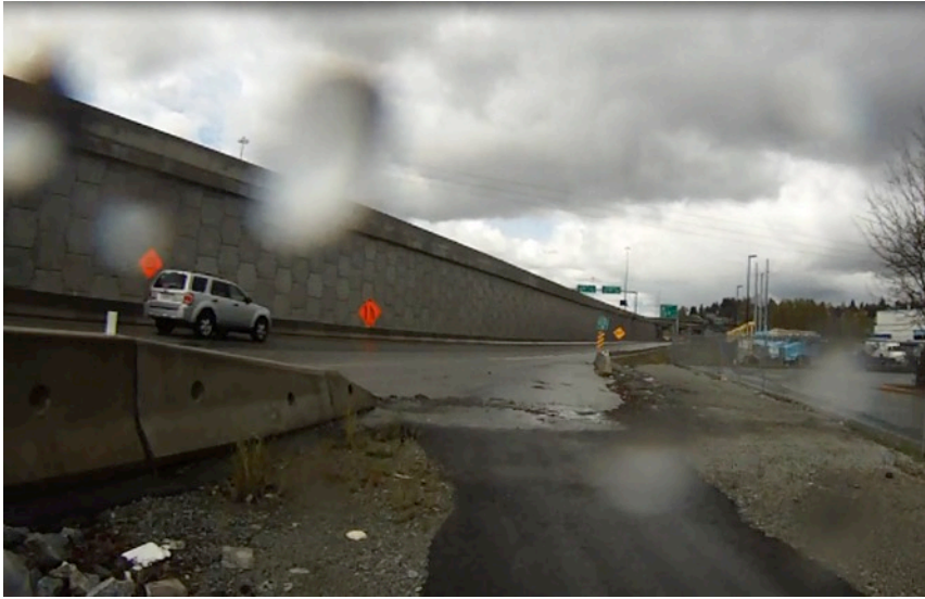
Missing protective bollards
