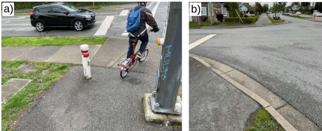
Figure 3. a) Angled curb drop at Deer Lake Ave and Waybourne Dr. Note that the bollard and light pole add to the
