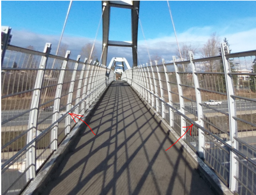
Figure 8: Bicycle Railing on Tynehead Overpass
